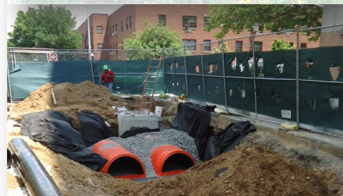
Underground Stormwater Chambers
